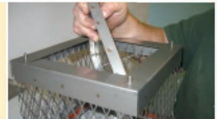
Angle damper and pull through frame, the flue is now ready for brushing.
