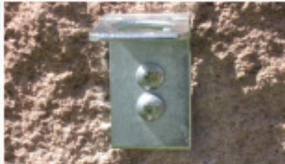
Hammer the tapcon and washer into the hole. Drill the lower hole and hammer in the second tapcon.
