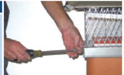
Tighten the screws on the cap-damper just like on a chimney cap.
