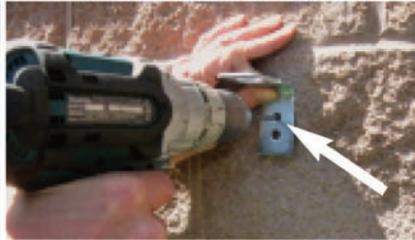
Position the firebox bracket about two feet above the firebox floor. Position in a convenient place for the customer to use. Drill the top hole using a 3/16" masonry bit.
