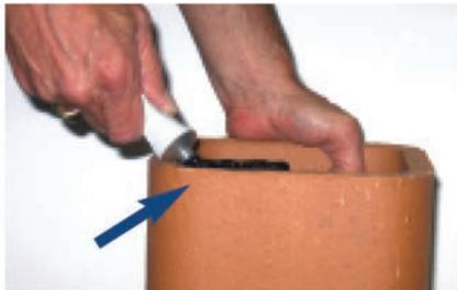
To achieve a total seal, first run a thick bead of silicone around the flue liner top.
