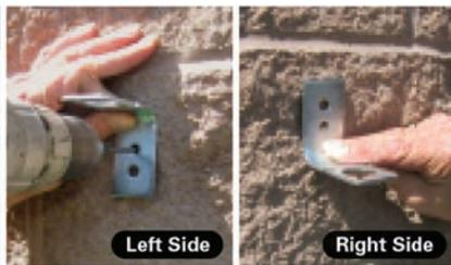
The slot in the firebox bracket should always be towards the rear. If placed on the left hand side of the firebox have the tail up, for the right hand side, tail down.
