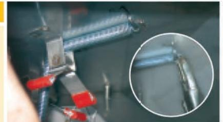
Release the bottom cable in the firebox. Remove damper lid and detach tension springs under lid.
