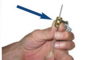
Fish the stainless steel cable from the smoke chamber and determine how much cable to cut off, leaving a few extra inches for future adjustments.
