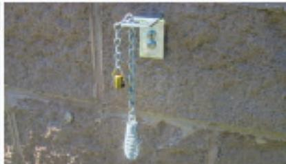
Thread the ball-chain assembly through the keyhole slot in the firebox bracket and let it hang.
